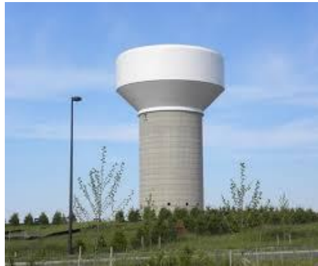
Water storage tanks are Typically, delegated designs
